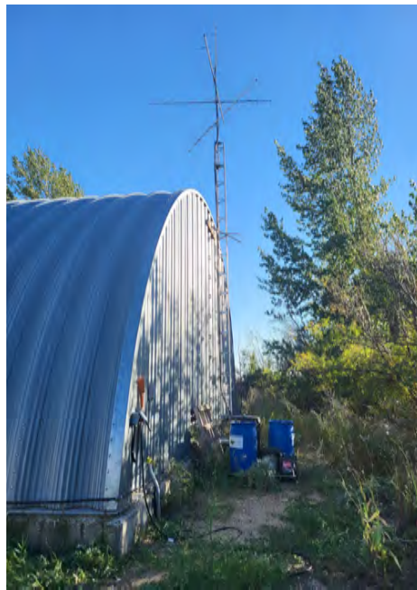
Motus tower at LMBO. Photo: Jordan Rustad
